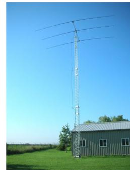
The basic antenna design is a narrow band design maximizing gain and front to back without regard to SWR bandwidth. The narrowband design has a natural impedance of about 22 ohms. Installed in the driver housing is a 50 to 22 ohm transmission line transformer Unun from the designs of Jerry Sevick W2FMI. The transformer has very low loss, less than 0.1 dB. I modeled the antenna using EZNEC on several bands. The
