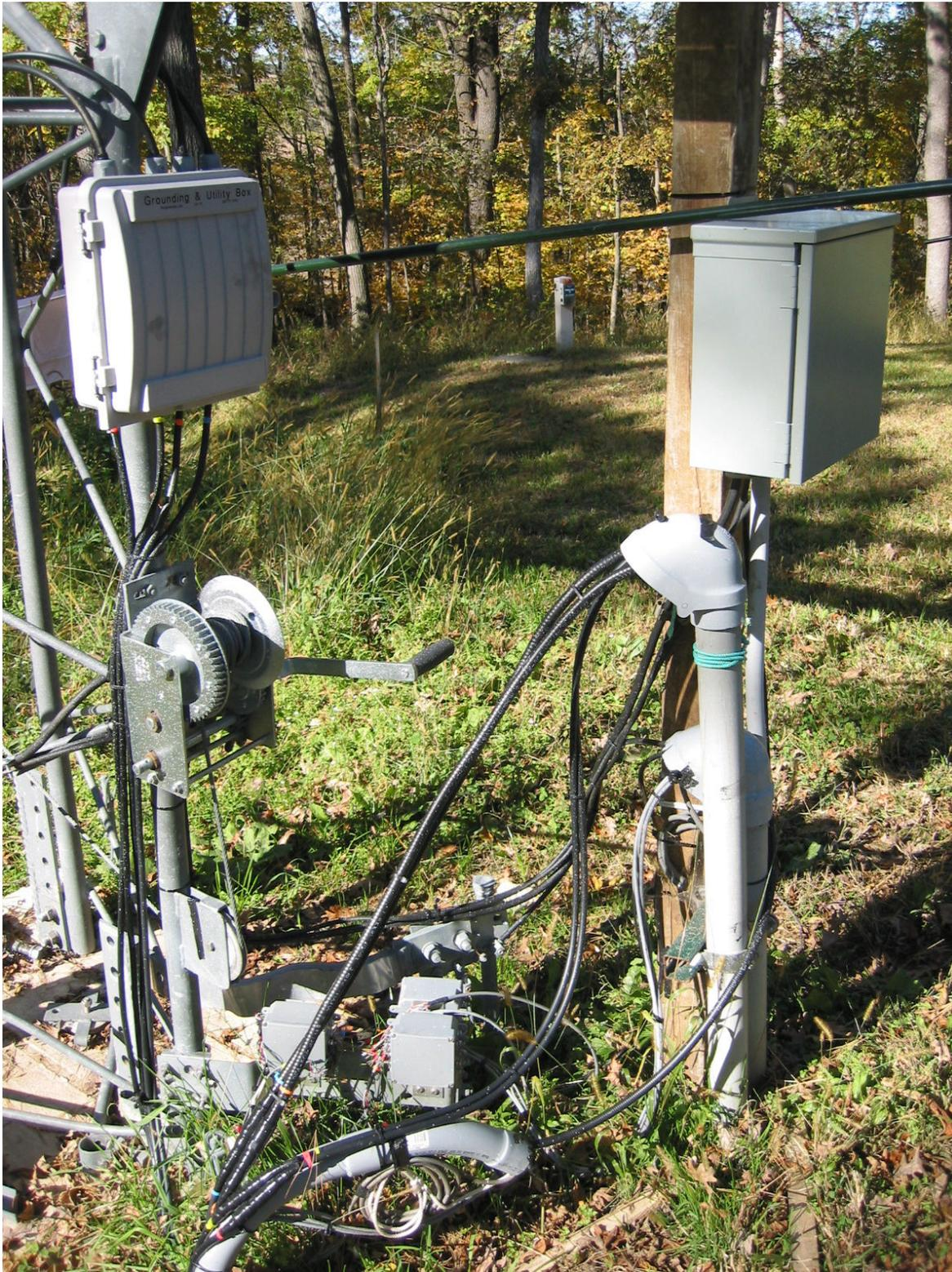
**#6:** The NEMA box on the left contains 4 Polyphasors for each of the 4 runs of coax/Heliac. The box on the right contains the LM470 motor control to raise/lower the tower. The two vertical PVC pipes are split into two: The tall one for the RF/coaxes and the lower one for the 40 control lines. The curved PVC at the bottom runs over to the base of the vertical phased array...about 50'.
