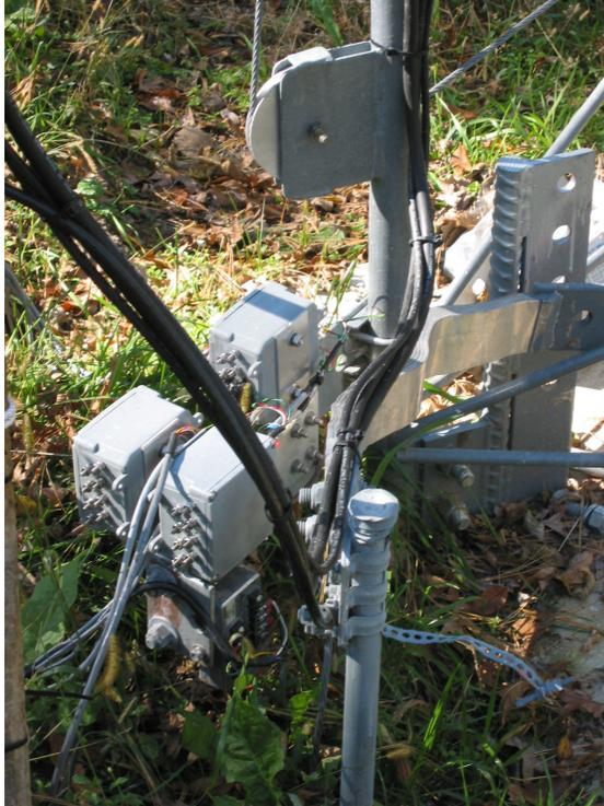
**#5:** This shows the grounding system at the base of the tower. The thick strap runs to that vertical 1" copper pipe. From that there is a #2 copper wire running under ground in a loop to 3 other copper stakes. There is also a #2 copper wire running from here to the house mains and the station ground.
