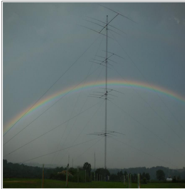
The main tower: 170' Rotating Rohn 55G with 4-el 40M and three 4-el SteppIR's.
