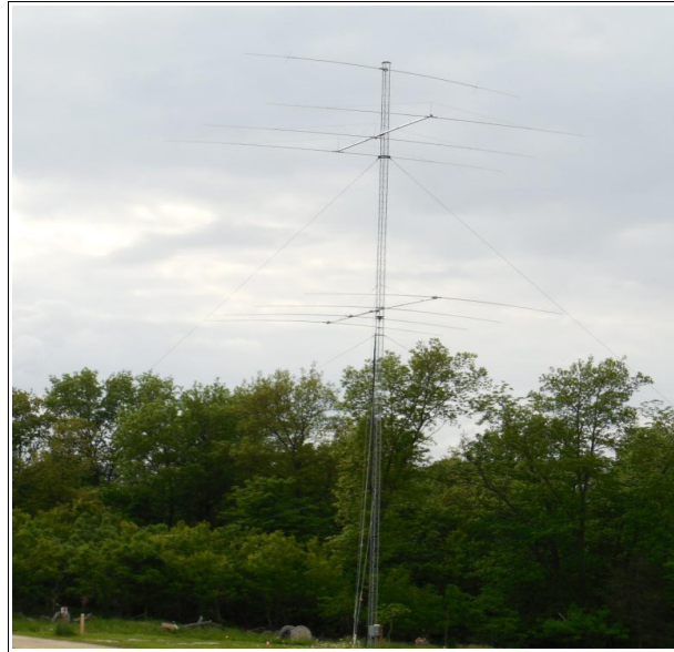
115' rotating Rohn 25G with 40M dipole, 3-el 30M and 4-el SteppIR
