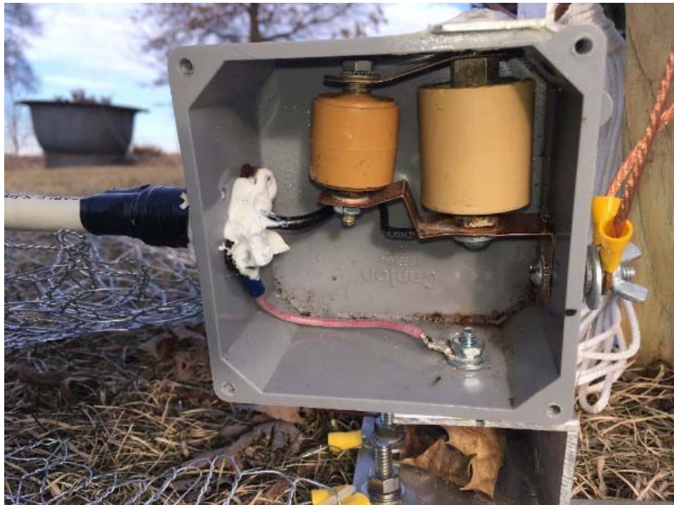
Feed is straightforward. The coax feeds direct to the screw terminal on the right (40/80). The two capacitors are in series with the 160m terminal (aluminum angle at top of box).
