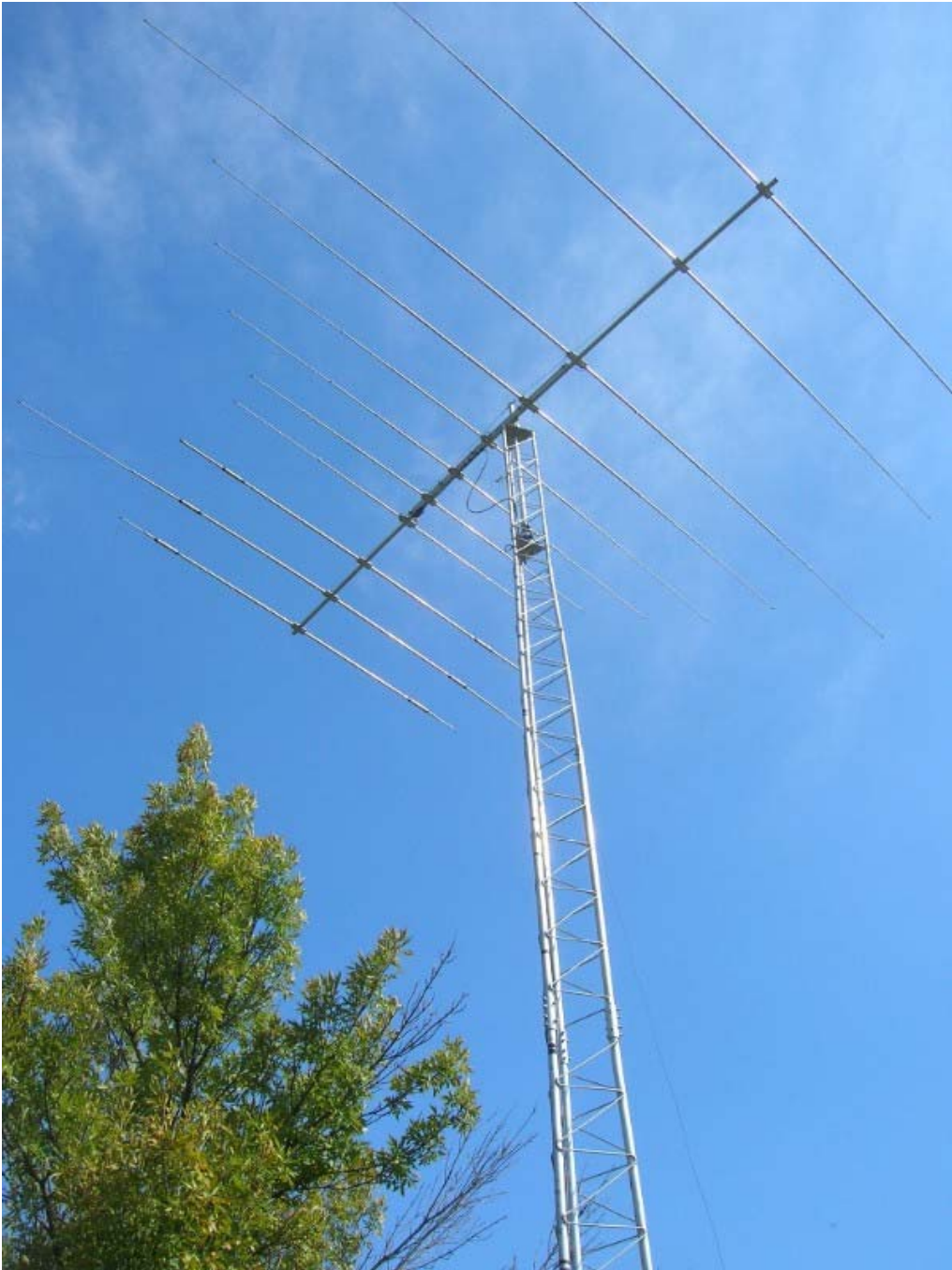
The TH-11 was erected in 1996, and it has performed very well.
