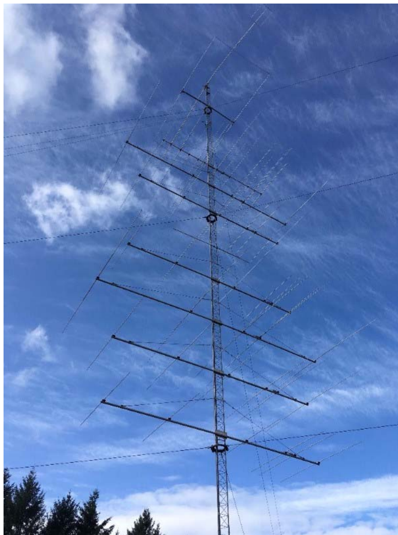
Antennas include: stacked monoband beams on 20/15/10, a 40m Moxon and 80m rotating dipole on the top (145')
