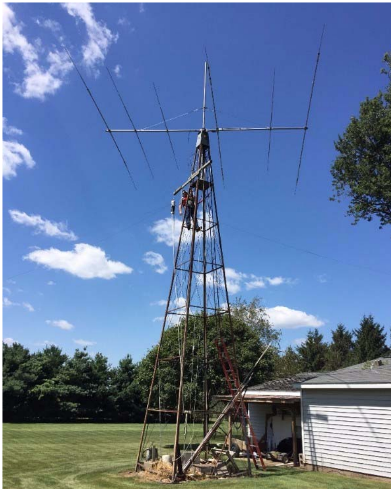
A nice day for a little antenna work - WØGXA
