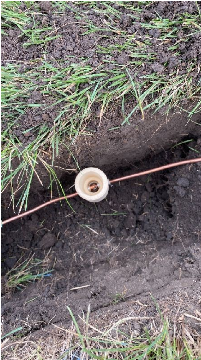
Cadweld set up to load
