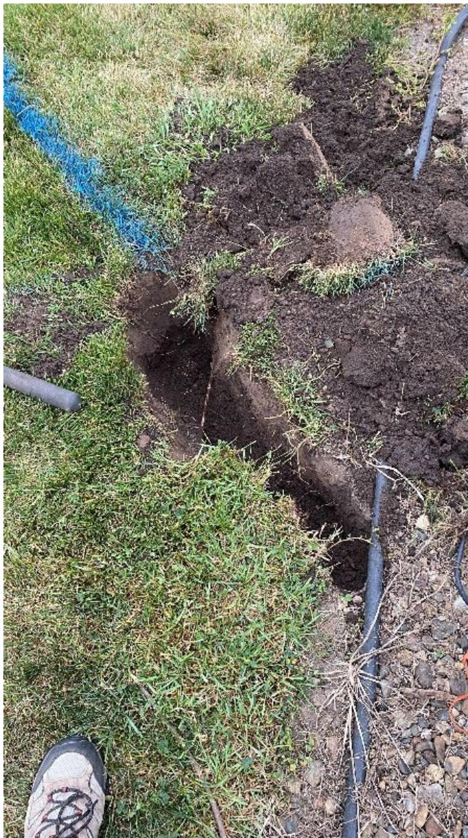
First step was the find the ground system around the windmill
