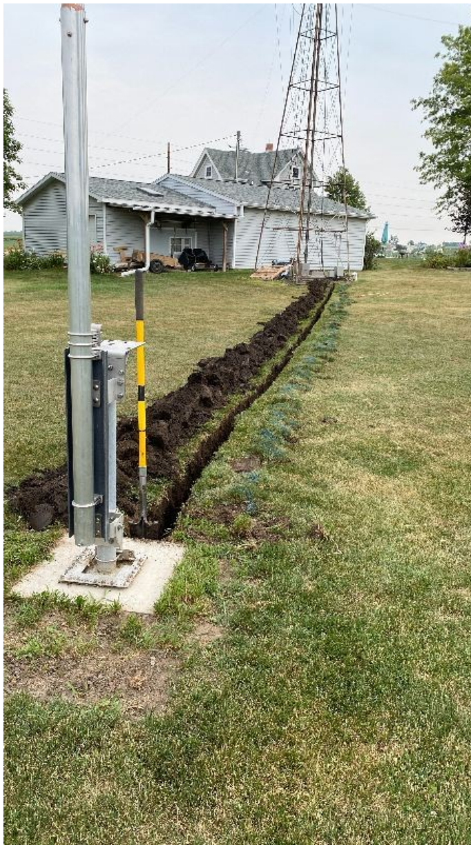
Digging is a lot like work but a tile spade is a very handy shovel to have on hand (makes the digging "easier").
