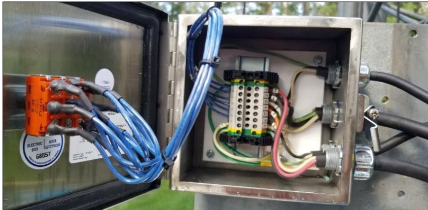
Tower Control Box AFTER:
